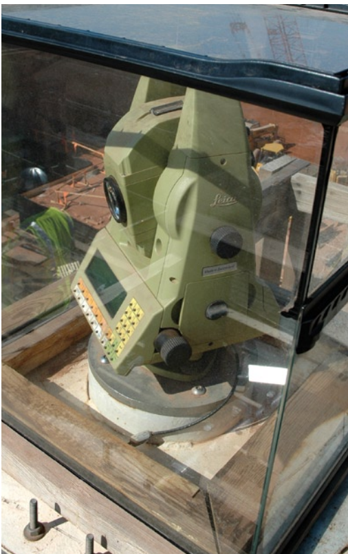
Top & bottom: Converted terrariums from a pet supply store proved to be the perfect on-site enclosures for the TCA1800 total stations.
