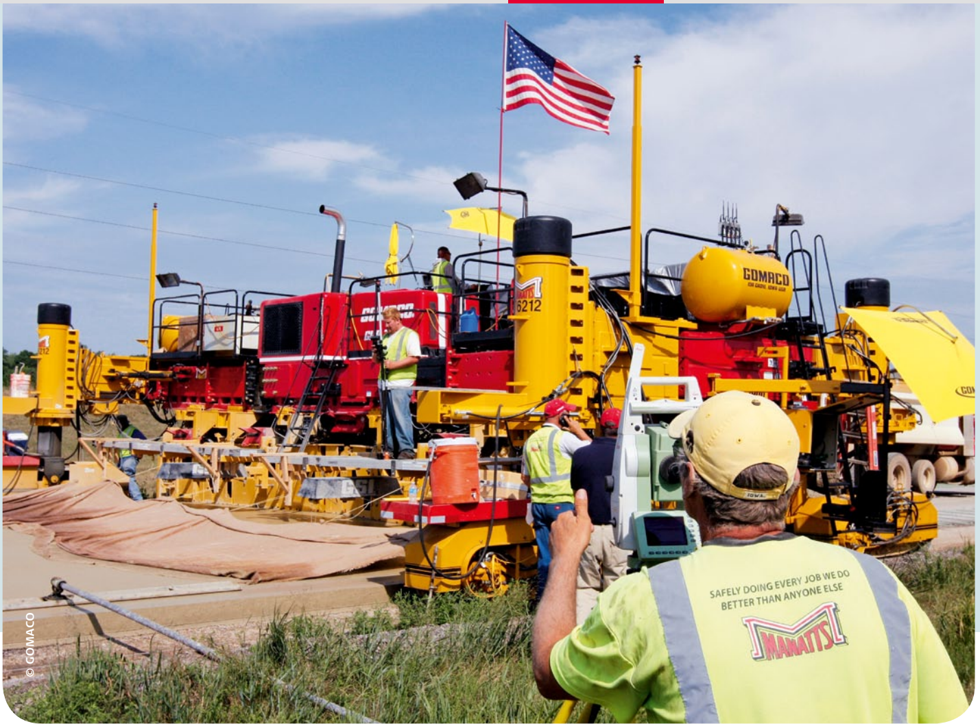
■ A crew member checks elevations on the new concrete surface with a Leica Geosystems total station.
